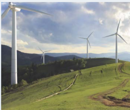
Wind turbine generator
